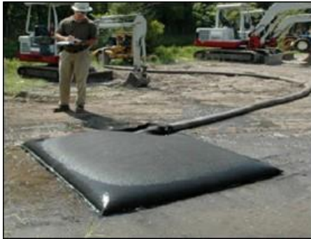
Plate 4-3 Silt Bag with water being pumped through
