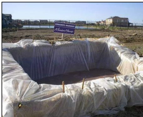
Plate 3-1 Typical concrete wash out areas
