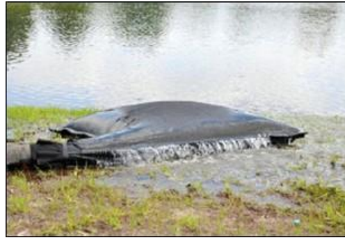
Plate 4-4 Silt bag under inspection
